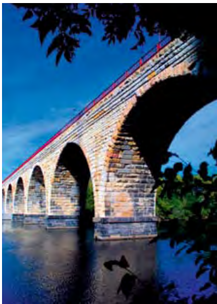
The Stone Arch Bridge was originally a railroad bridge. (Meet Minneapolis)
