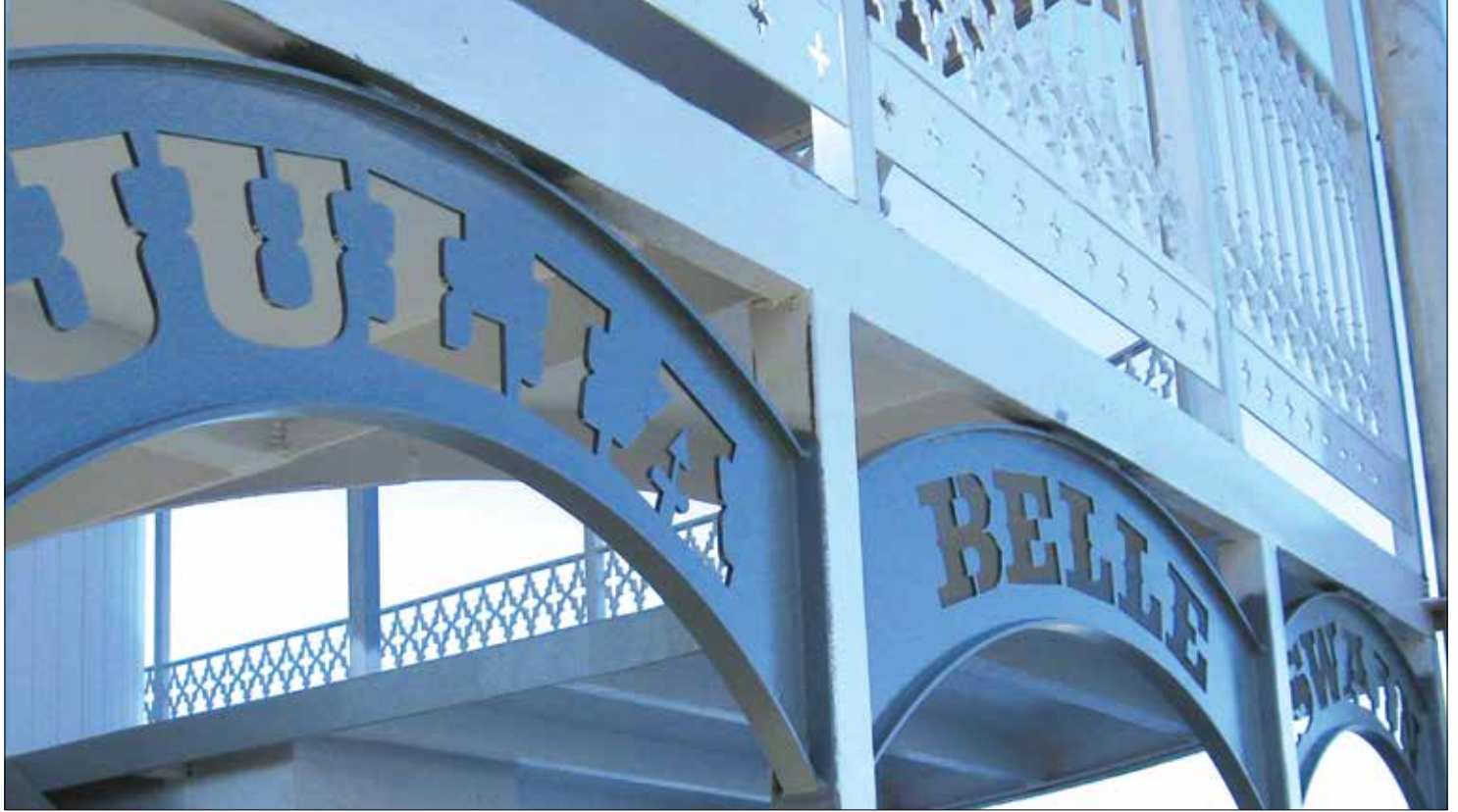
New aluminum arches will welcome passengers about to climb the main salon stairway.
