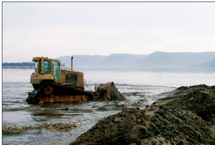
Island building is serious work, but it sometimes looks like big toys playing in the mud. (Army Corps of Engineers)
