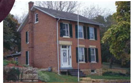
The first Grant home has been restored as a private residence. (Galena Public Library)
