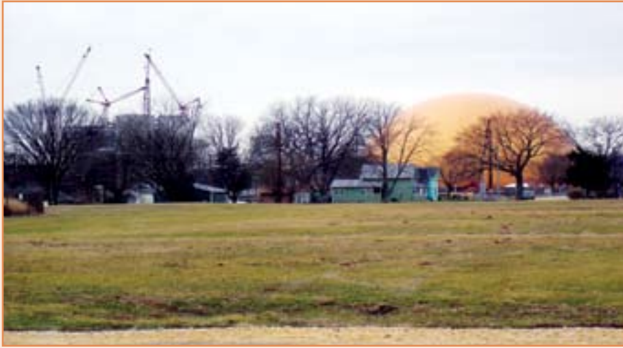
ADM Clinton's coal storage dome glows behind South Clinton houses. (Julie Johnson)
