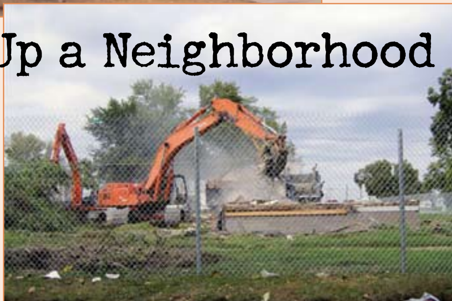
A backhoe claw tears apart a South Clinton building. (Dixie Foster)
