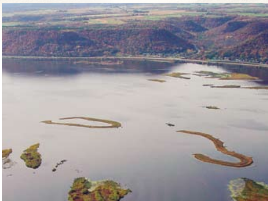
These two islands in Pool 5 were constructed with sand dredged from the Main Channel. They are designed to collect more sand in their "shadows" downstream. (courtesy Army Corps of Engineers)
