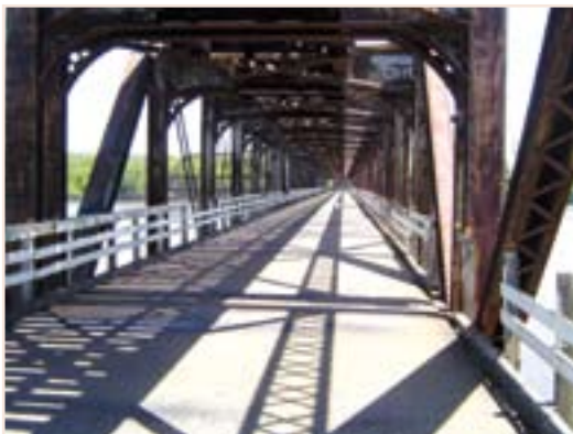
Half of this abandoned swing bridge could be made into a fishing pier extending from Inver Grove Heights, Minn. (Dakota County)
